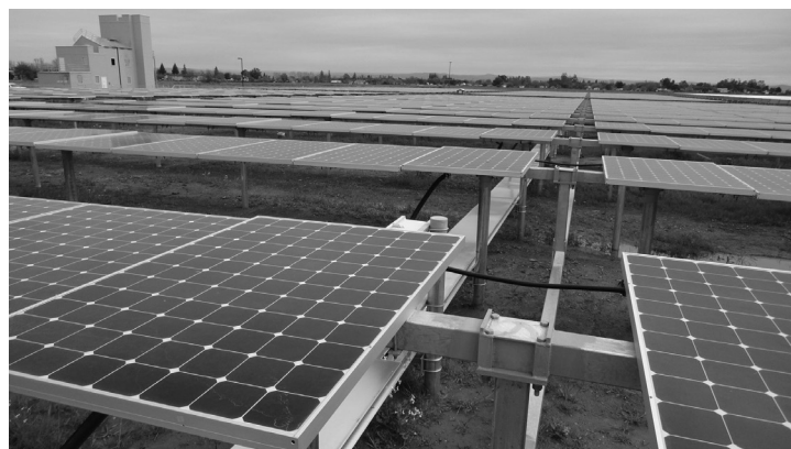
The photovoltaic field on campus helps to reduce energy consumption.
